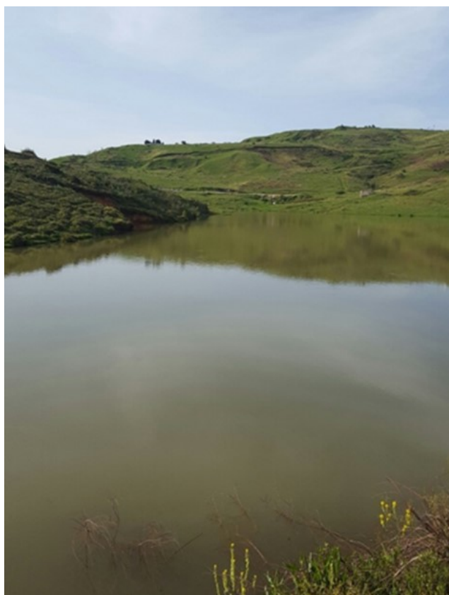
FIGURE 1 A view of study area, the Al-Bireh Dam, Syria.
